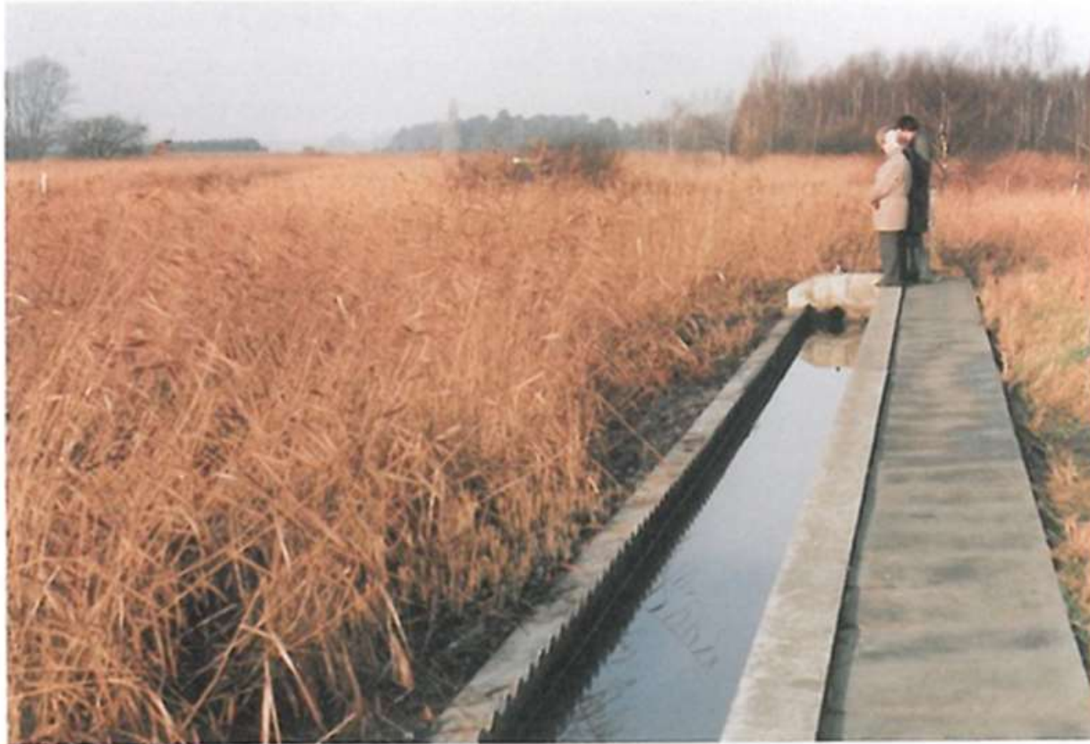
Fig. 1. Inlet channel and reed bed on the Southern works after 10 years operation
